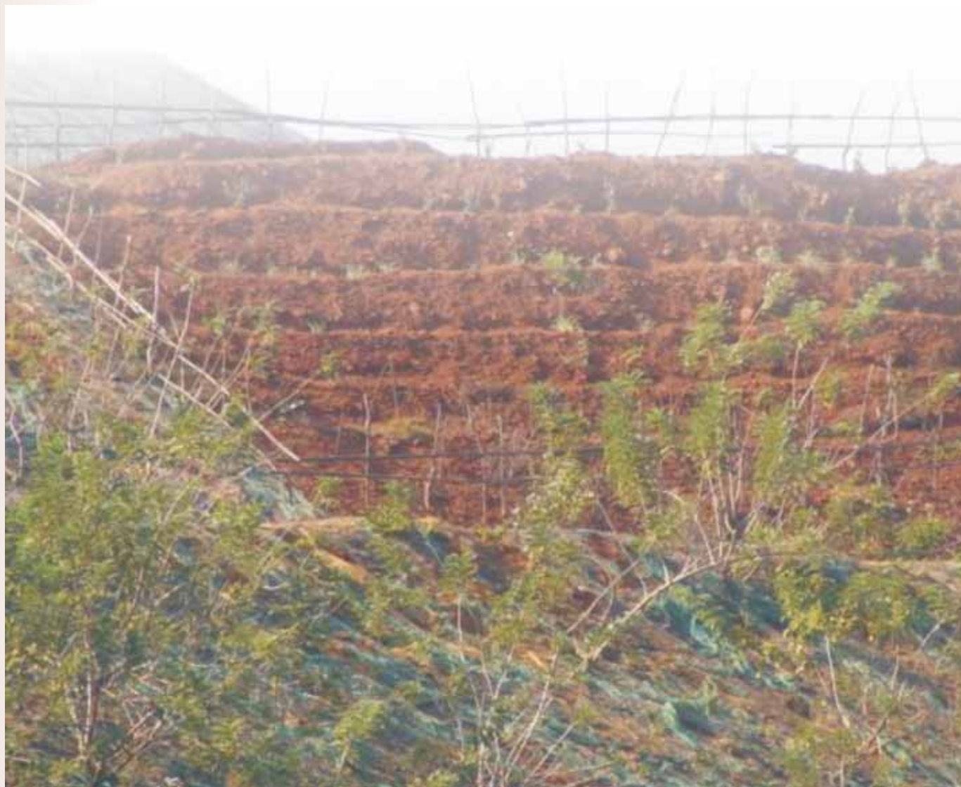
Plantation on waste dumps after terracing at Codli Iron Ore Mine
